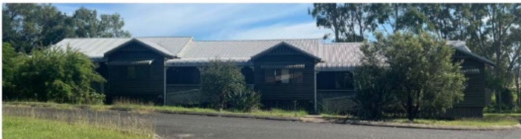
Exterior of Building comprising units 1, 2 and 3:
